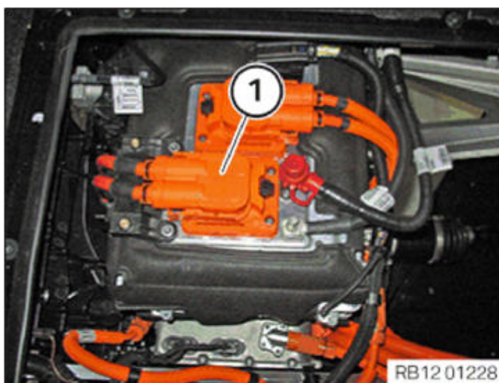
Fig. 315: Identifying High-Voltage Cable Courtesy of BMW OF NORTH AMERICA, INC.
